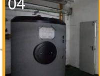
Hot water tanks installed to the buildings (capacity of 5 m³ at a temperature of 55-60 °C), in order to store the hot water produced by the hybrid heat pumps and the solar panels.
