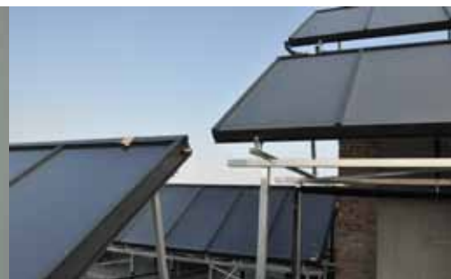
Solar collector system
