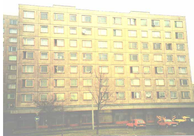
The SOLANOVA building before refurbishment.
