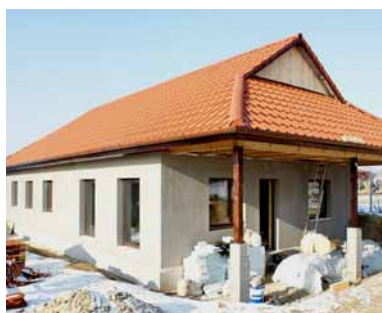
Passivhaus in Szada just before commissioning.
