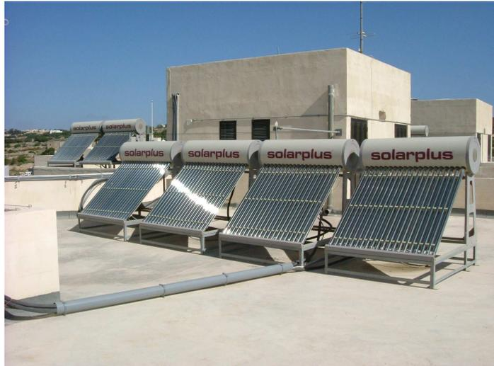
**Figure 2: Solar water heating systems installed on the roof of the Sustainable Housing Project at Tal-Ftieh, Birkirkara, Malta.**
