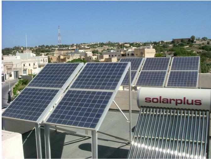
Figure 3: The 1.5 kWp Photovoltaic system, comprising 10no. modules and an inverter, connected to the showroom of the Housing Project.
