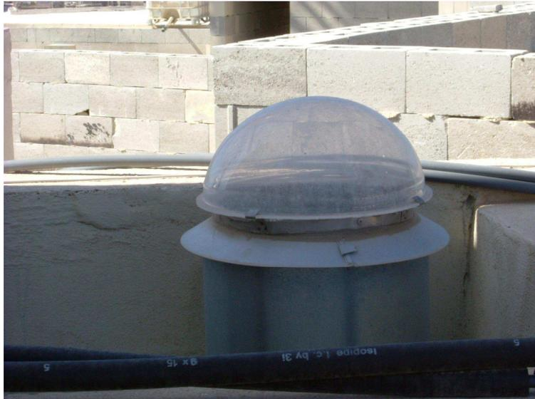
Figure 4: One typical sun pipe installed and capped at roof level, running down through the shaft to the underlying garages at basement level.
