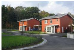
The Swedish residential area Vallda Heberg aims at reaching the national passive haus standard for its buildings. The standard includes specific construction elements in the building design, including air tight envelopes and supply and exhaust ventilation with heat recovery. [Read more](#)
